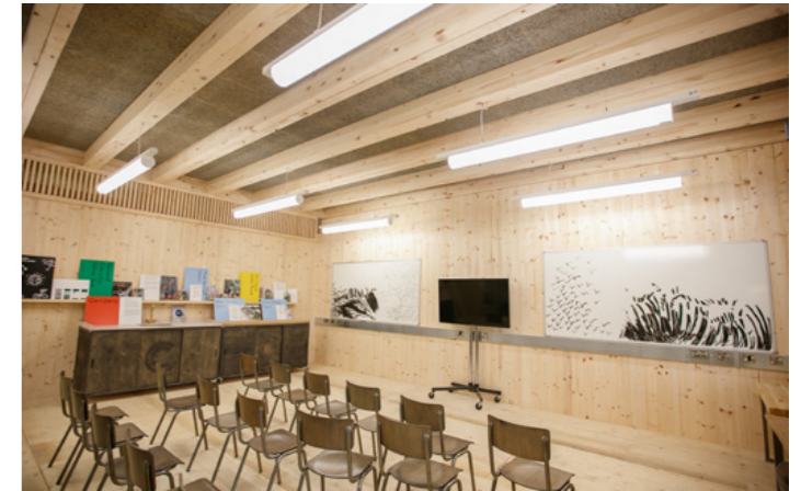
Figure 4. GenZero classroom. Manufactured at BE-ST from homegrown CLT and Glulam. Photo: BE-ST
